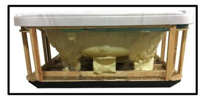
Deactive the power to the spa. Remove the old skirting and measure the height. The new skirting will be installed the same way or butting up to the shell
