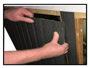
Starting at the left flange install the first panel as shown using three of the color matched screws.
