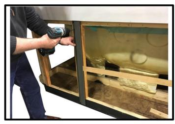
Using three screws in each flange, install both flanges onto each of the 2x4's used to frame out the service opening.
